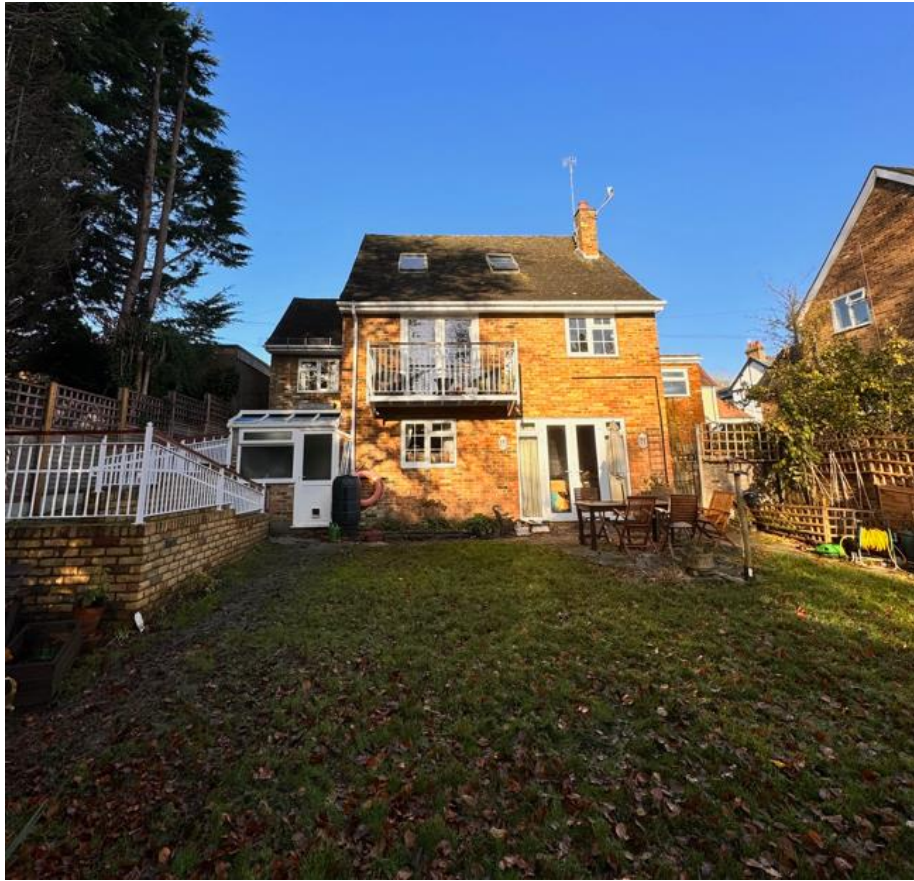
Figure 5 Existing Rear Elevation
